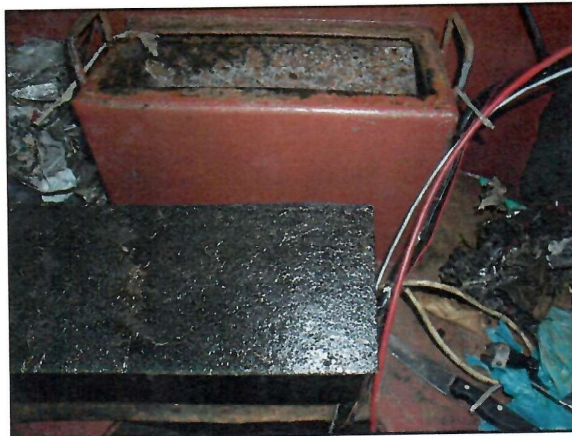
Weed hatch with cover removed.
