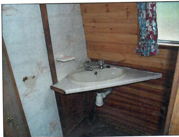
Bathroom showing the corner hand basin.
