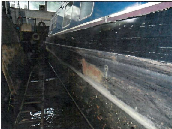
Hull sides showing scuff marking.
