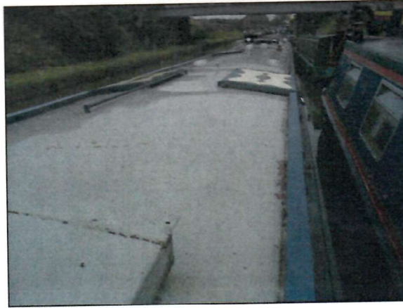
Cabin roof showing deteriorated paintwork.
